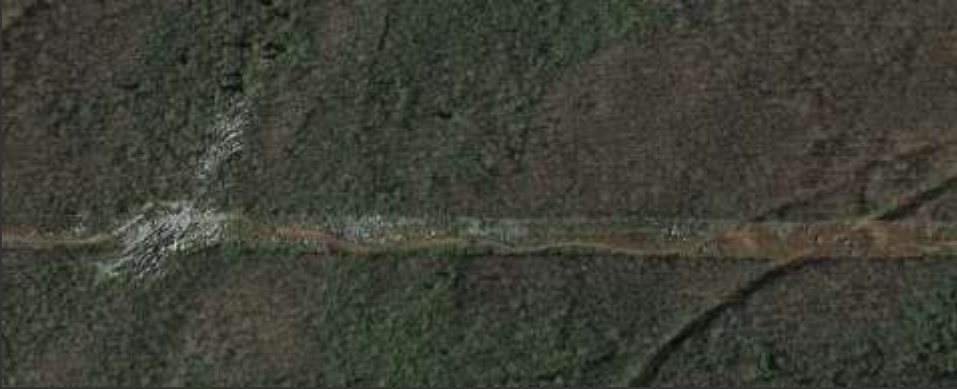
Example: Electrical transmission line in Tucker County, West Virginia (Google Earth)
