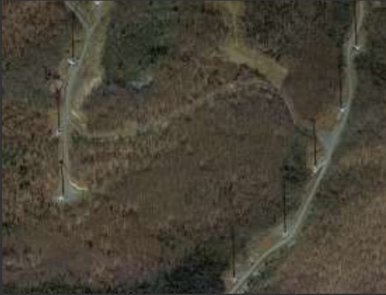
Example: Wind Farm in Grant County, West Virginia (Google Earth)
