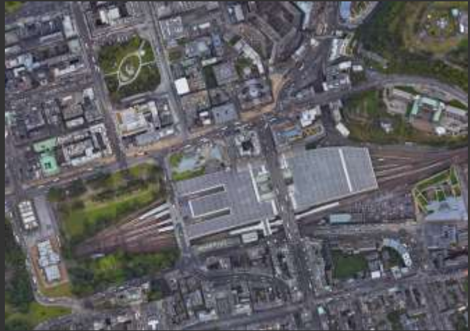
Example: Train Terminal in Edinburgh, Scotland (Google Earth)
