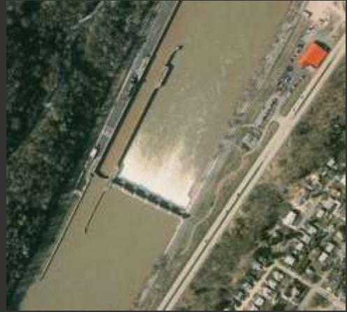
Example: Lock and Dam on Monongahela River in Morgantown, WV (Google Earth)
